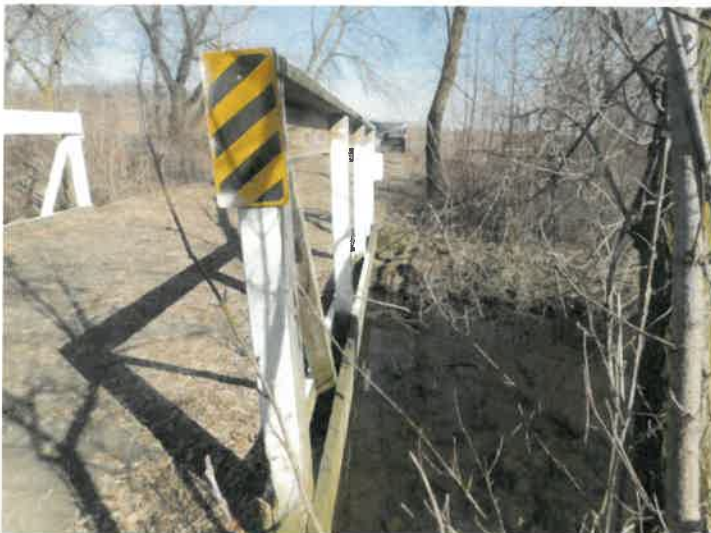
Photograph #2 – snow mobile bridge, SE corner
