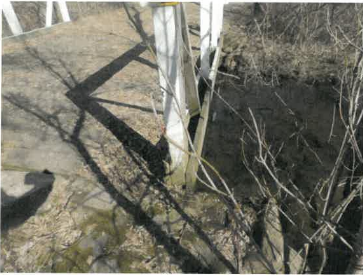
Photograph #1 – snow mobile bridge, SE corner
