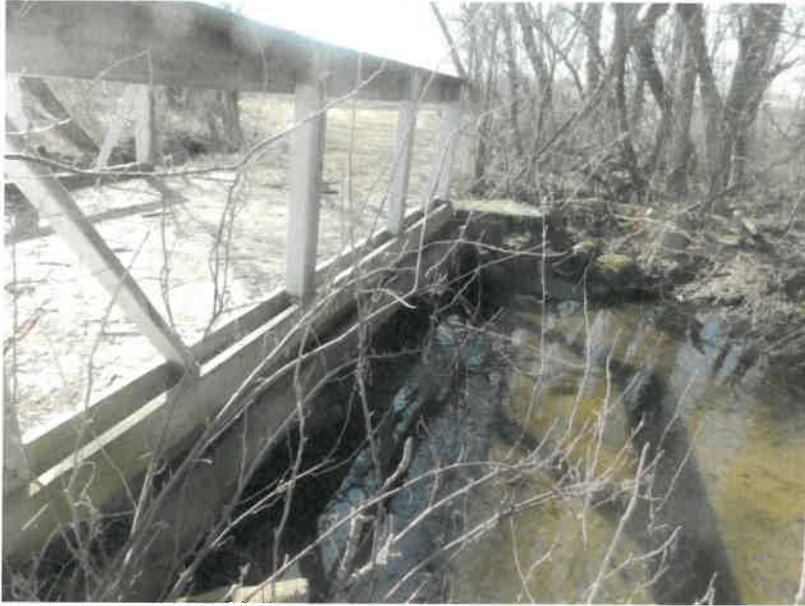
Photograph #5 – snow mobile bridge, NW corner
