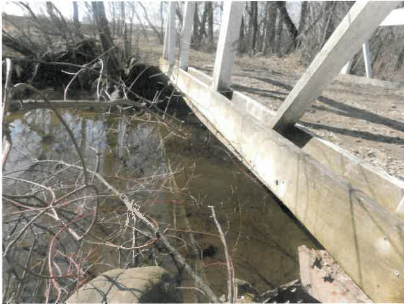
Photograph #7 – snow mobile bridge, NE corner
