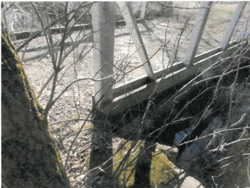
Photograph #4 – snow mobile bridge, NW corner
