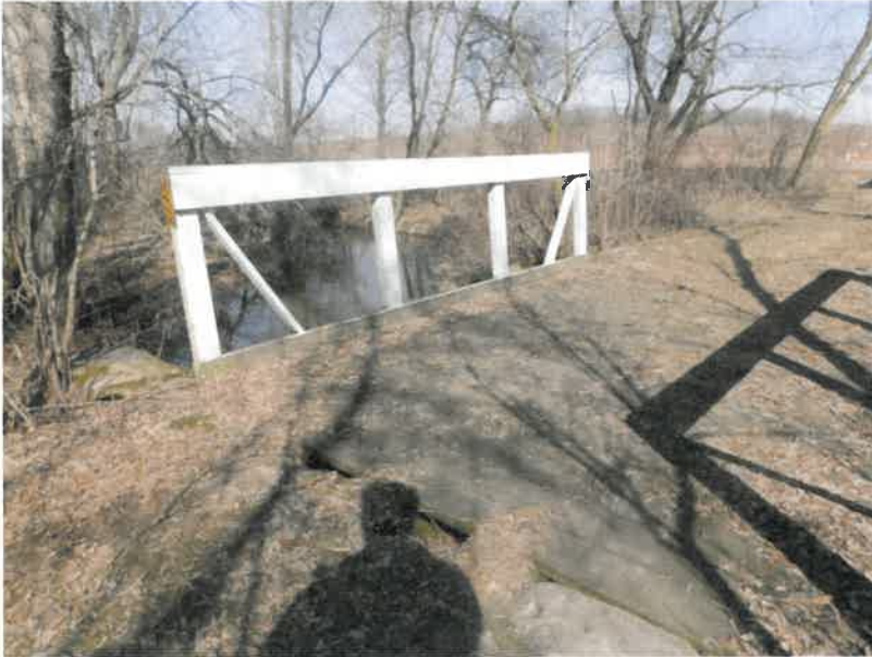
Photograph #3 – snow mobile bridge, SE corner
