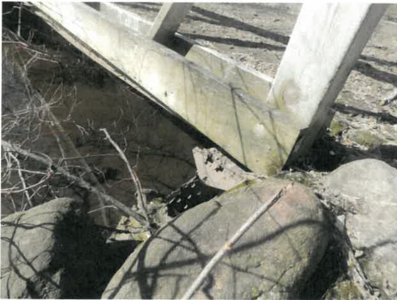
Photograph #6 – snow mobile bridge, NE corner
