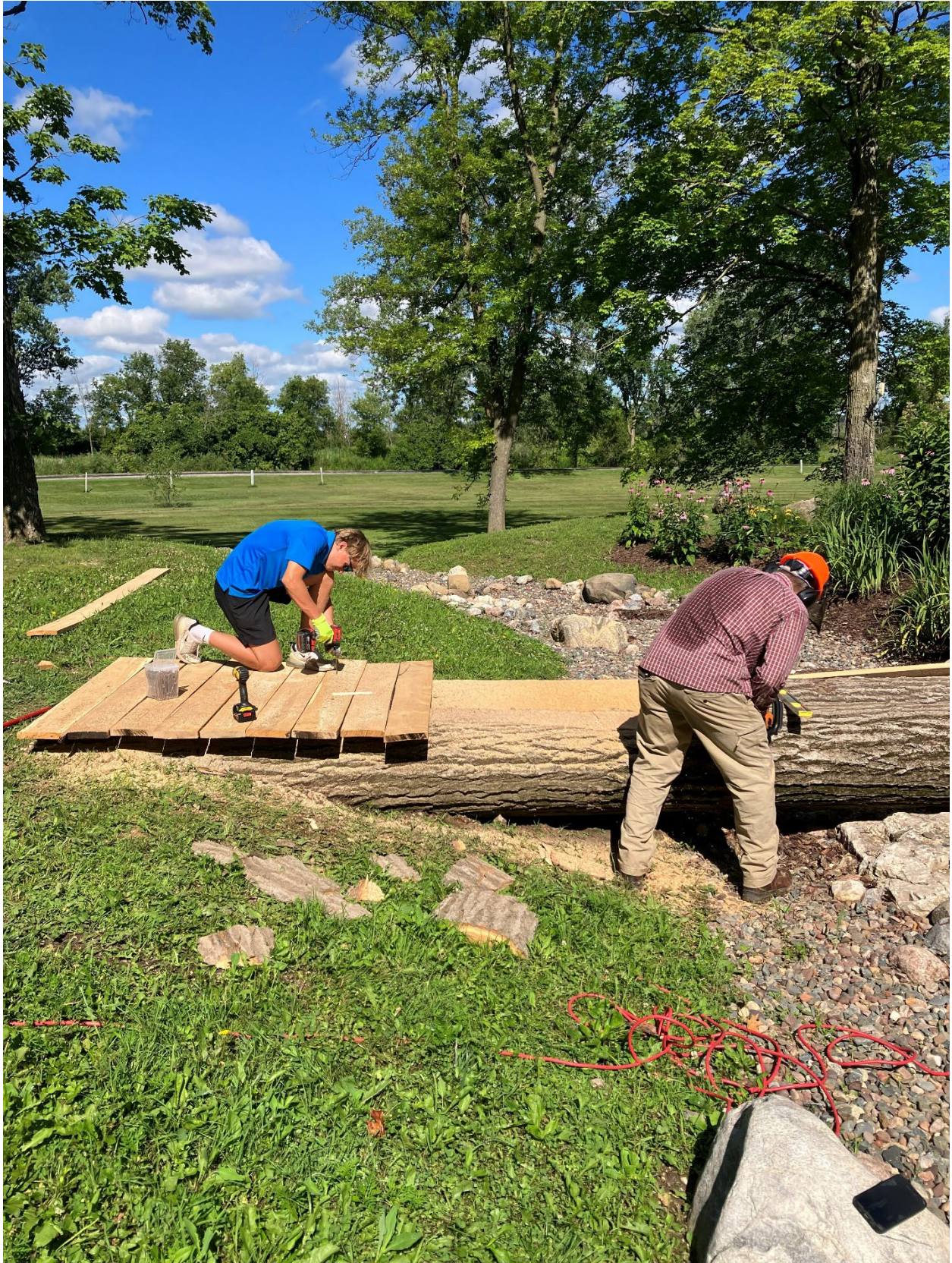
Figure 42 - Kohler Center for Marsh Education Landscaping Work July 2025
