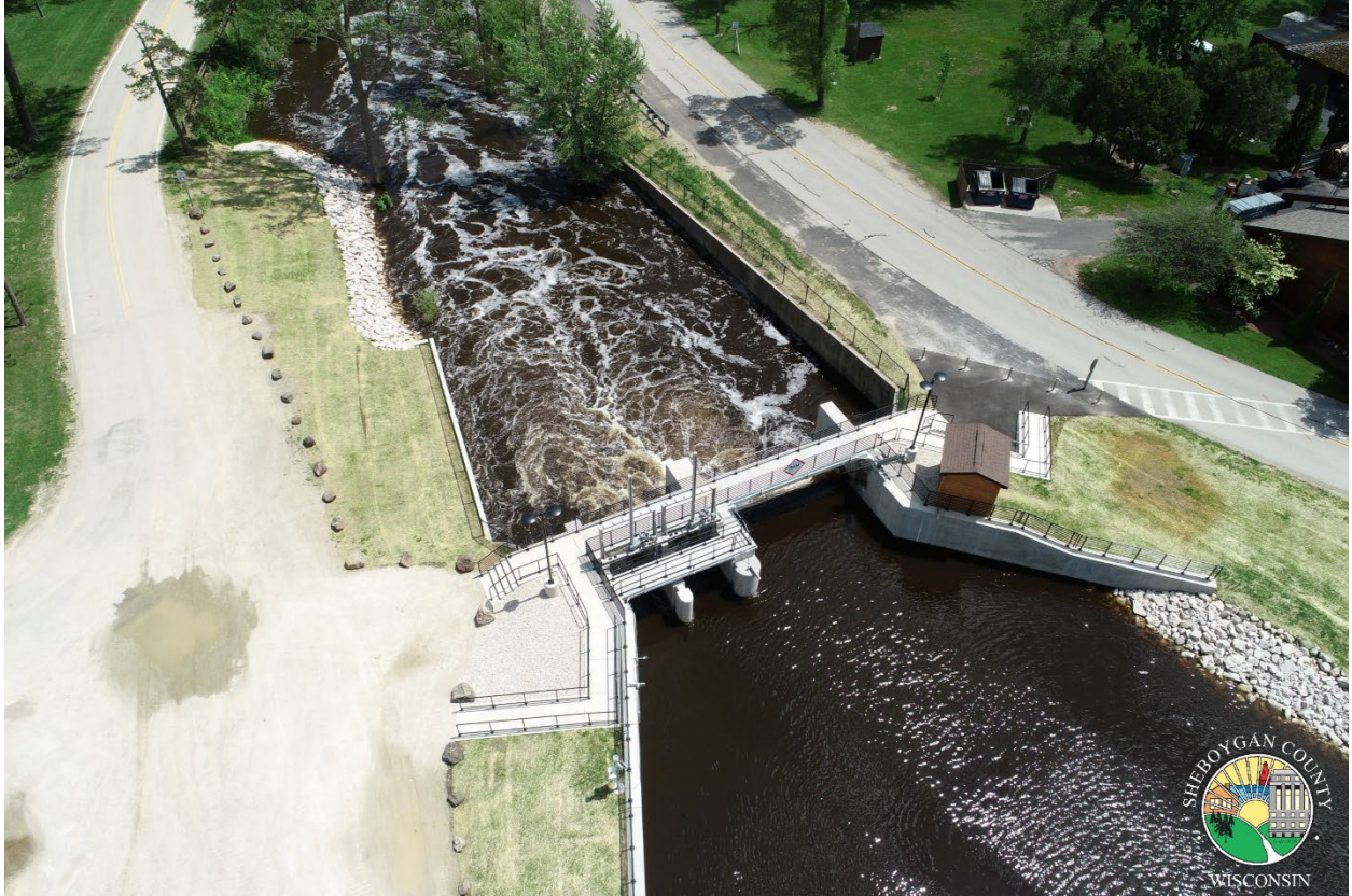
Figure 38 - Completed New Dam May 2024
