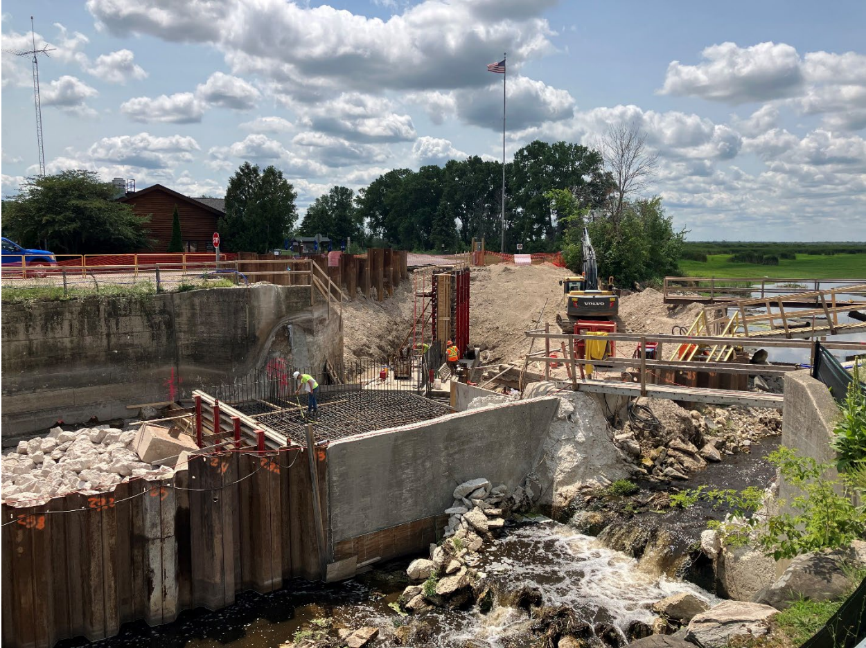
Figure 37 - Early Stages of New Dam Construction June 2023
