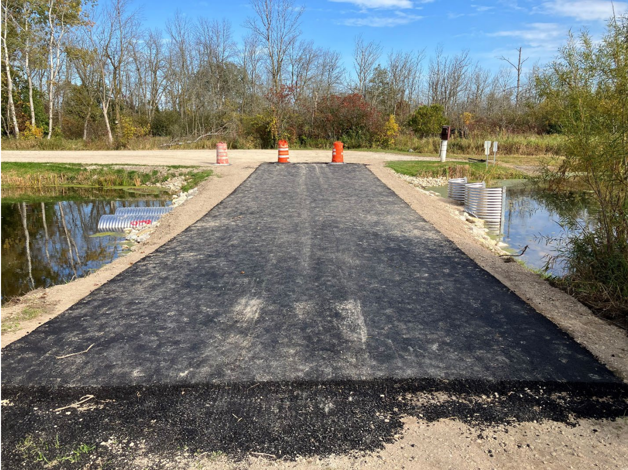
Figure 39 - New South Ditch Xing and Control Structures 2022
