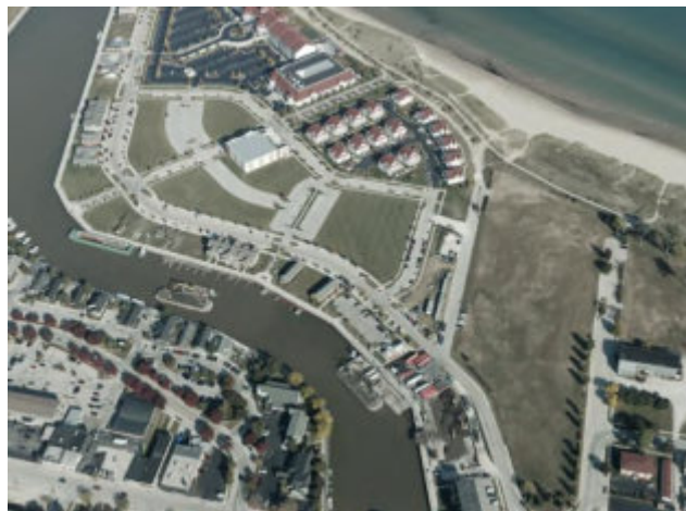
Sheboygan River Harbor During Dredging Period
