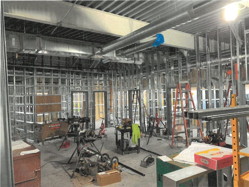
INTERIOR STUDS COMPLETED
