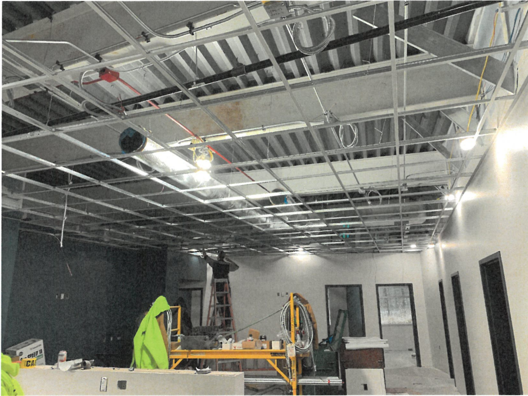
DRYWALL, PAINT & CEILING GRID
